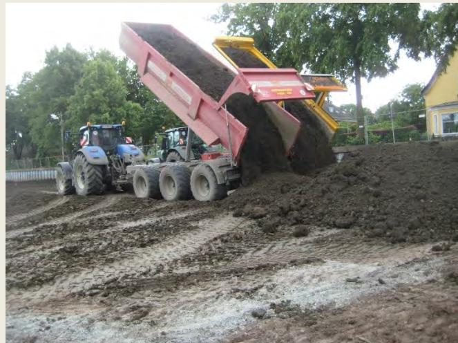
**Figure 39 : dredging spoils as building material**
