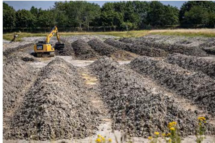
**Figure 25: Bremen-Seehausen: dredging spoils on the dewatering fields**
