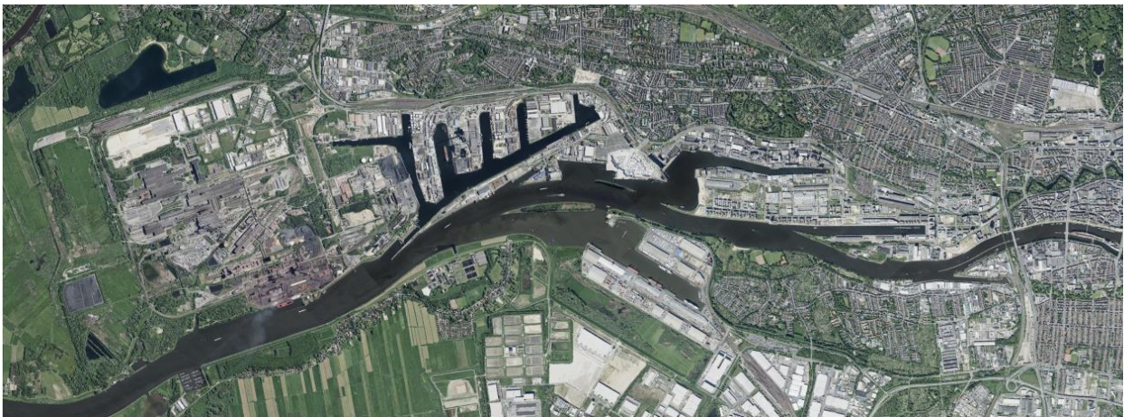
Figure 8: Aerial picture of the “Industriehafen” and the “Neustädter Hafen”
