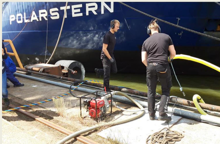
Figure 28: Preparations for inwater-cleaning on a biocide-free hard coating
